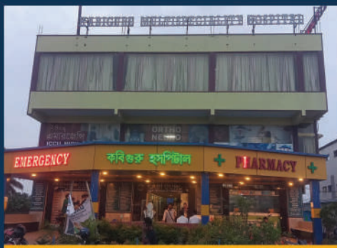
Kabiguru Multi-Speciality Hospital
